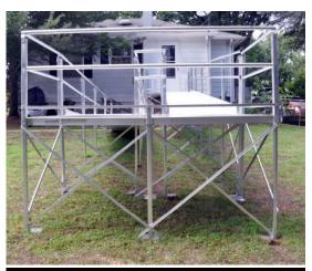
Lower end of brace should be within 6 inches of ground. Anchor footplates securely to ground.
